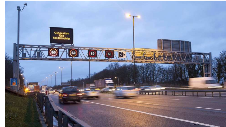
M4 Smart Motorway
